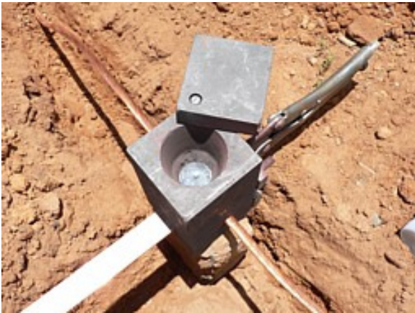
The top block is clamped on and the tin disc is inserted first. Powder is added on top. A "fuse" powder leads fire into the block.
