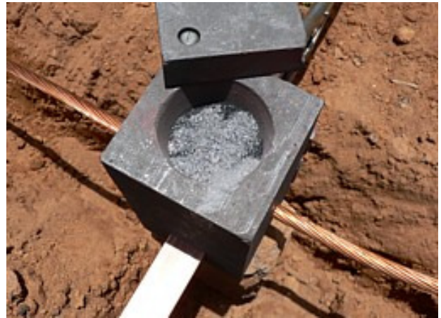
The top block is clamped on and the tin disc is inserted first. Powder is added on top. A "fuse" powder leads fire into the block.
