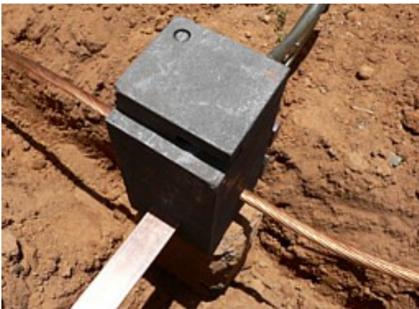
Firmly closed with the fuse powder showing. Light the powder and POOF - enormous heat amalgamates the tin and copper. See p1.
