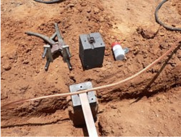
Hardware: Bottom and (inverted) top block, clamp, magic powder and circular tin disc. Note: block is specific for bar and wire size.
