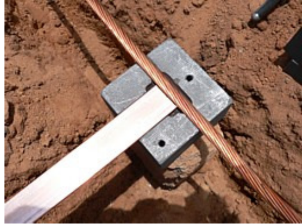
Hardware: Bottom and (inverted) top block, clamp, magic powder and circular tin disc. Note: block is specific for bar and wire size.
